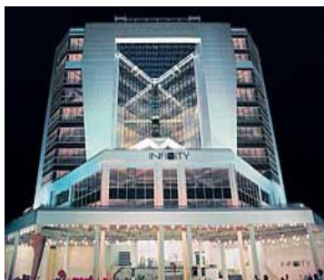
An IT building in Sector V
