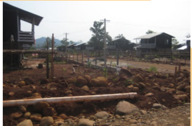
Condition of Housing in Resettlement Zone After Displacement
